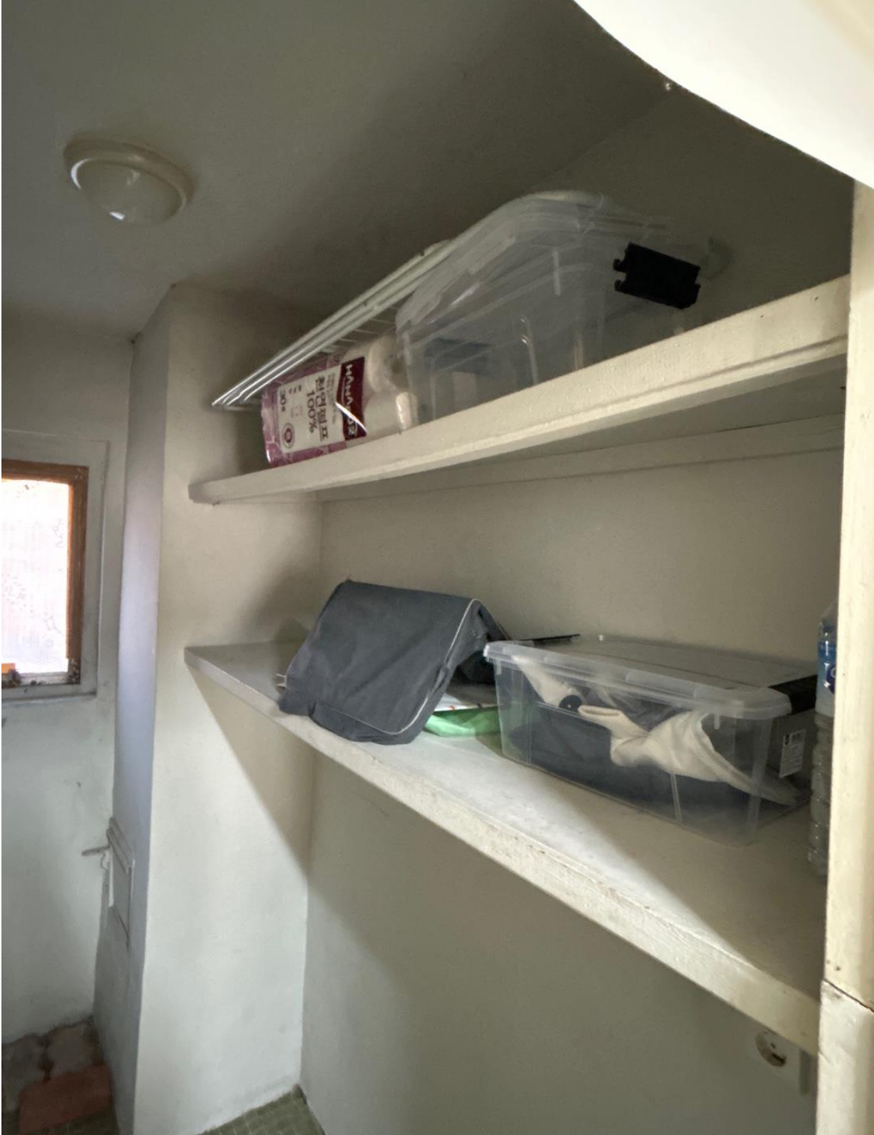
Multipurpose room (used as storage)
